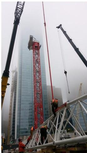
In good hands: Experienced Maxim Crane Works service technicians, thoroughly trained by WOLFFKRAN service experts, assembled the WOLFF 700 B in just three days. (Source: WOLFFKRAN)
